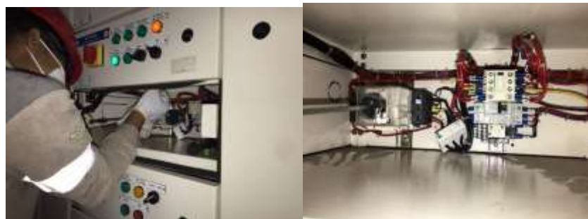
Gambar 16. Instalasi Sensor Energy
